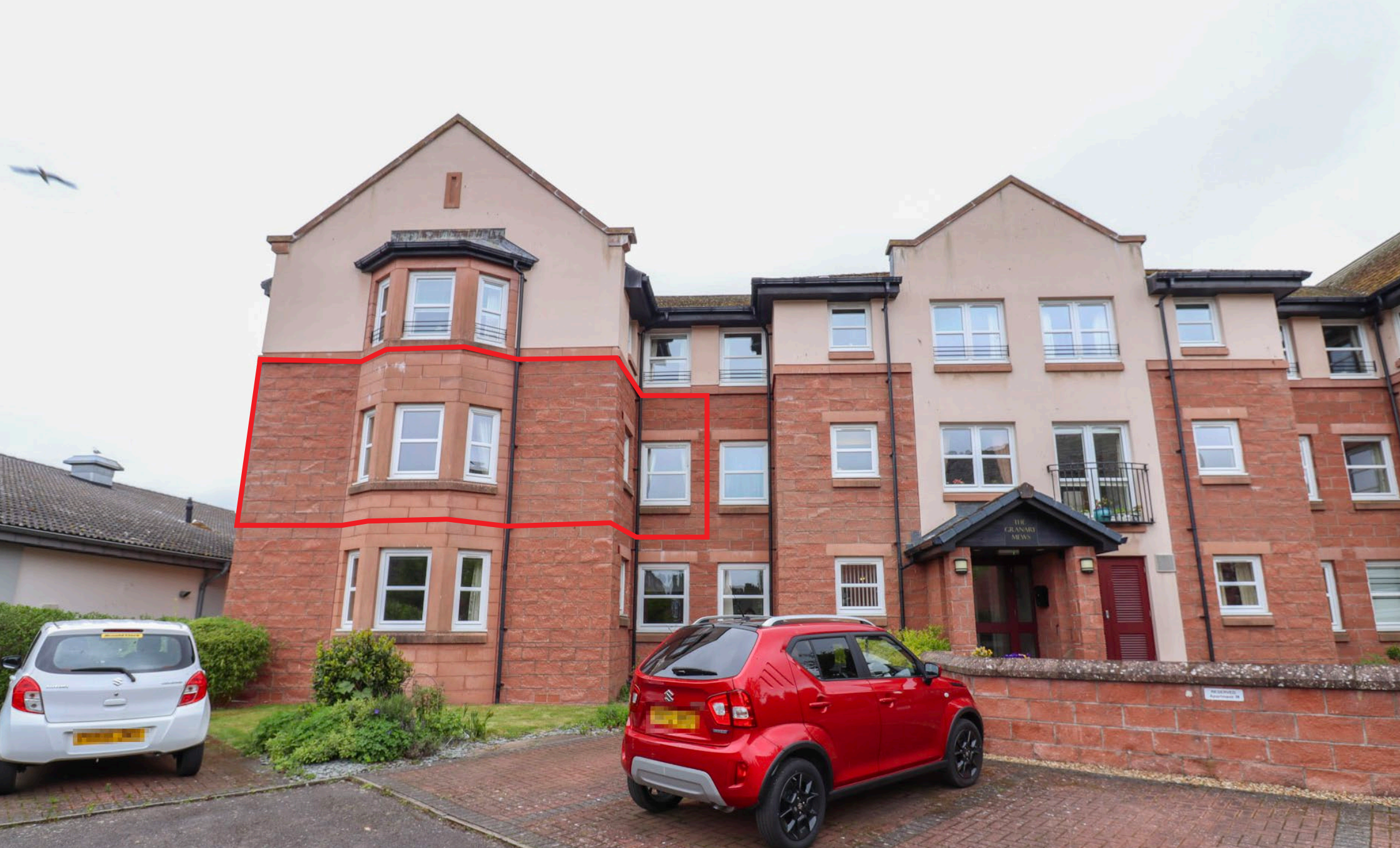
Flat 79, The Granary Mews, Glebe Street, Dumfries, DG1 2LU
